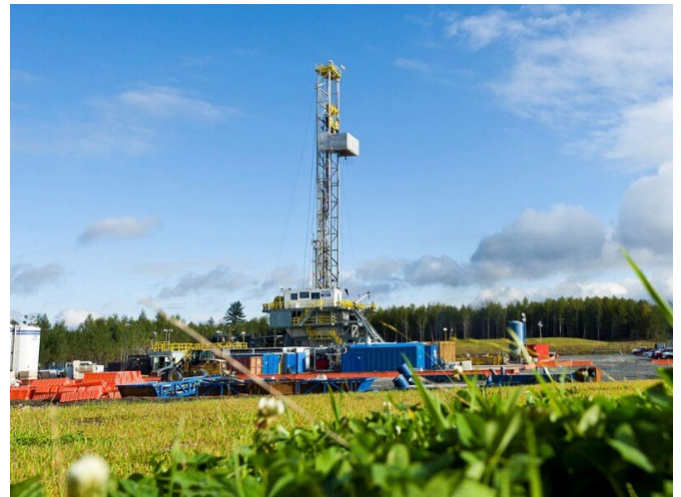
Sage Geosystems well work in Starr County, TX
